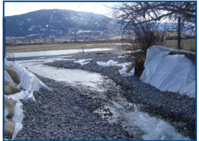
Figure 9. Conveyance channel constructed to reduce erosion from discharged pumped water.
